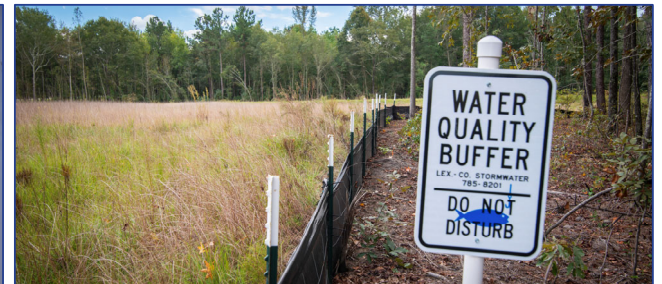
Silt fences and buffer areas protect surface water, groundwater and wetlands.
